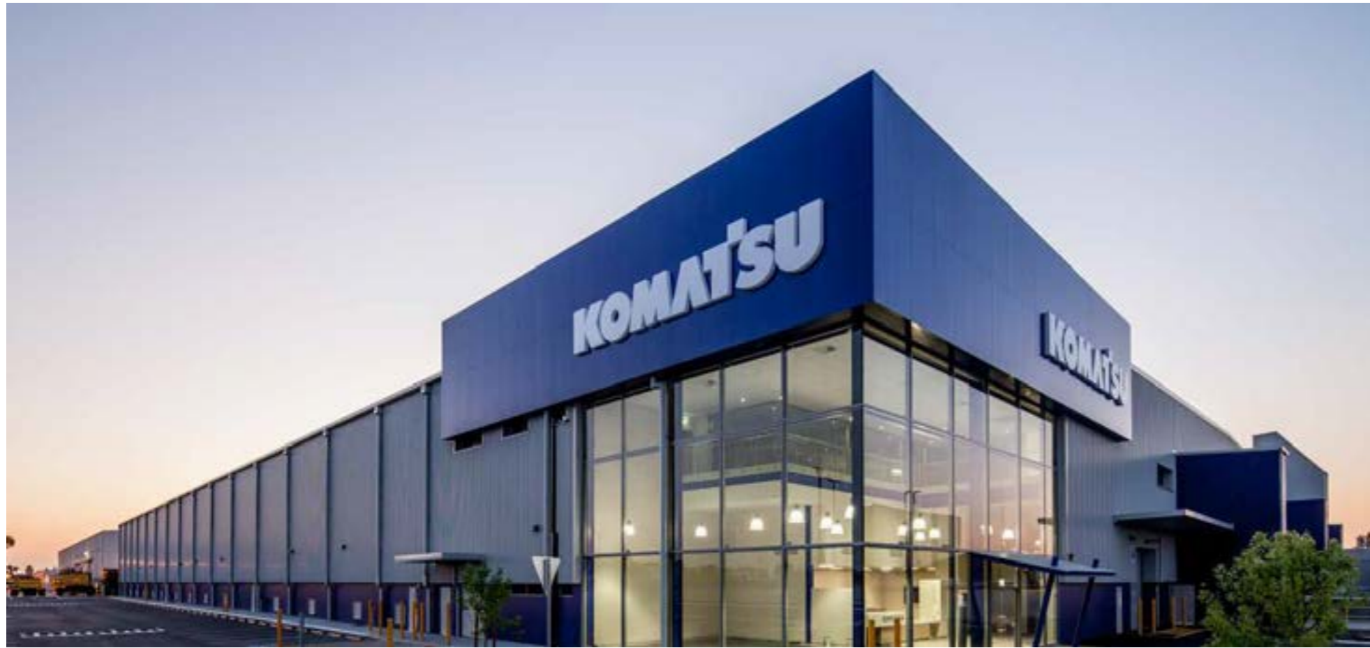
Welshpool Distribution Centre, Perth
