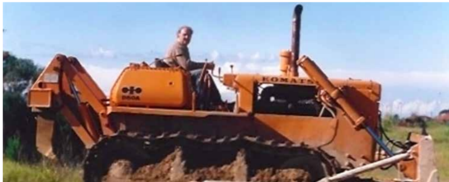
Bruce Leer operating the Komatsu D60A-6 dozer
