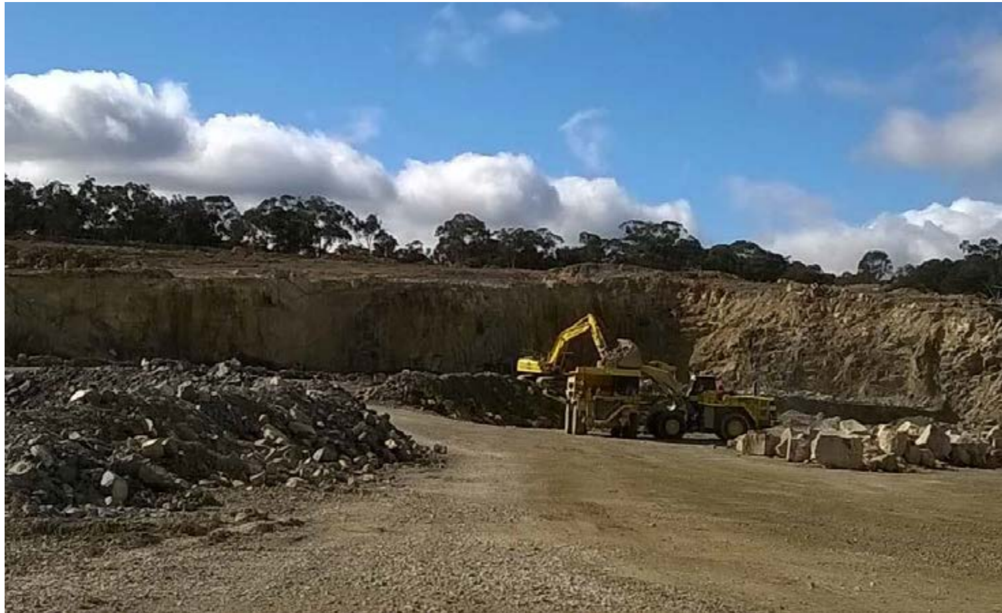
Holcim Lynwood worksite
