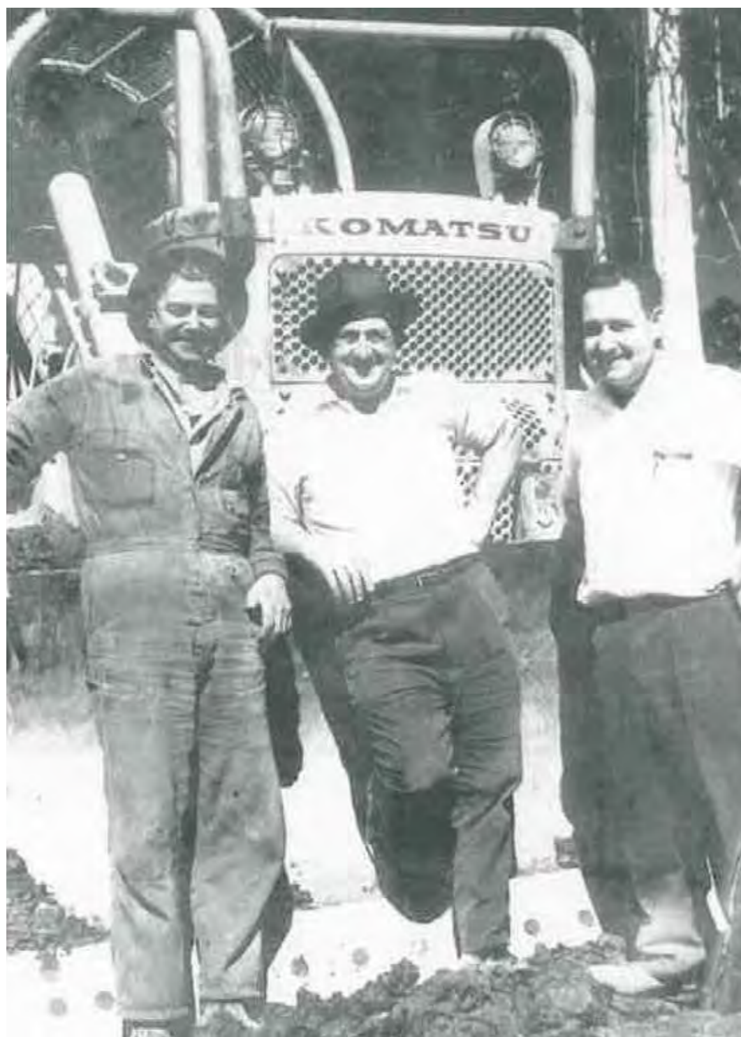
D80 Komatsu Dozer at the 1967 handover From left: Bert Stride, Bob McKenzie and Le Tourneau Westinghouse Service Manager, Stan Lynch
