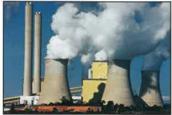
▲ NS Komatsu Gippsland Branch (brown buildings), dwarfed by the mighty Loy Yang power station.
