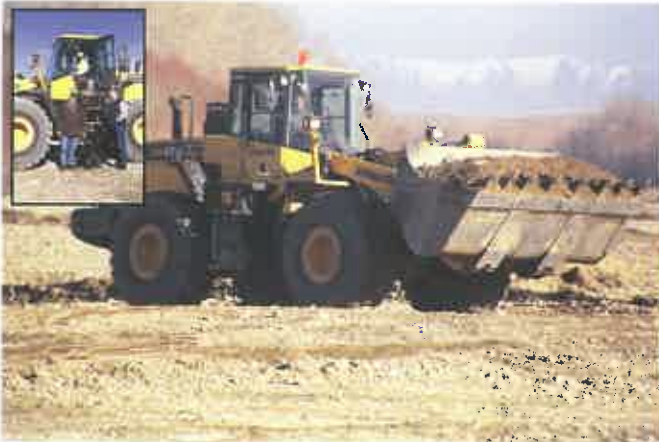
NZ's first Dash 5 loader, South Canterbury Screening & Crushing's WA470-5. Inset shows operator Steve Harliwich (in cab) with owner Paul Smith, and Komatsu rep Phil Thomson.
