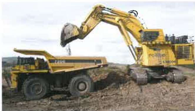
HWE's Komatsu PC4000 loading one of eight 730E dump trucks.
