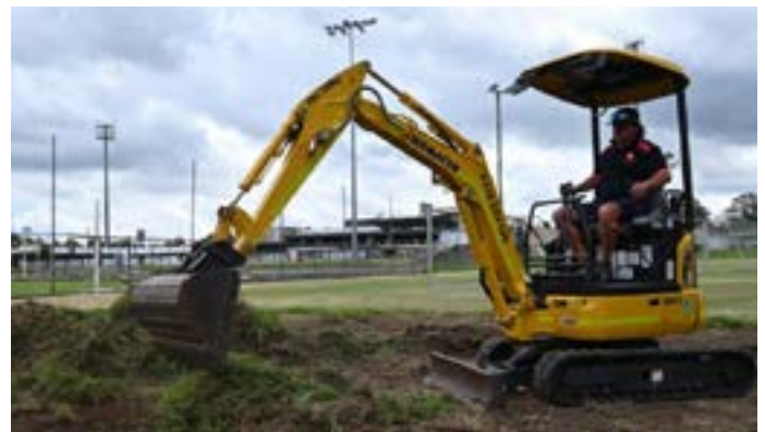
Pictured: Home ground remediation and repairs.
