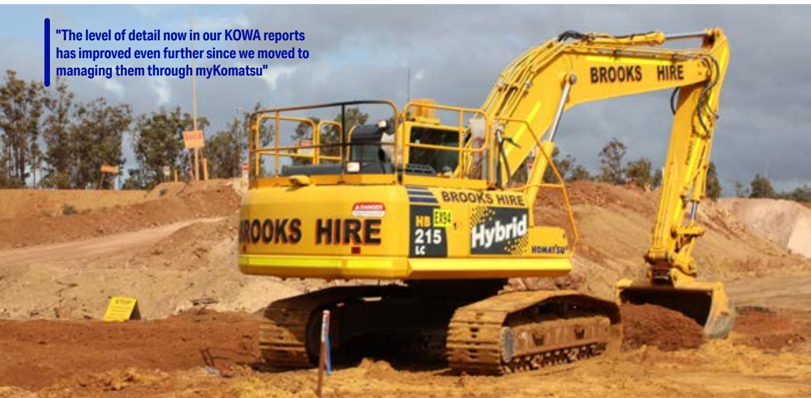
Pictured above: Brooks Hire's HB215LC Hybrid Excavator at work.
