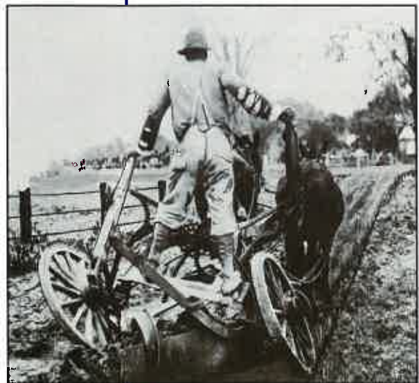
▲ The first leaning wheel grader, developed by J.D. Adams in 1885
