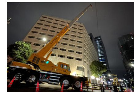
Trees being removed by crane
